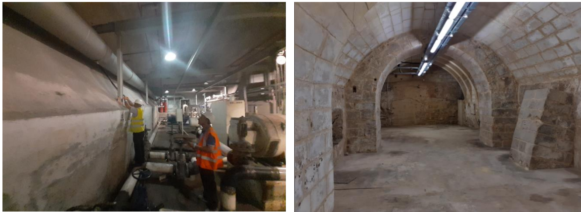
Figure 4 Examples of the subterranean work areas.
